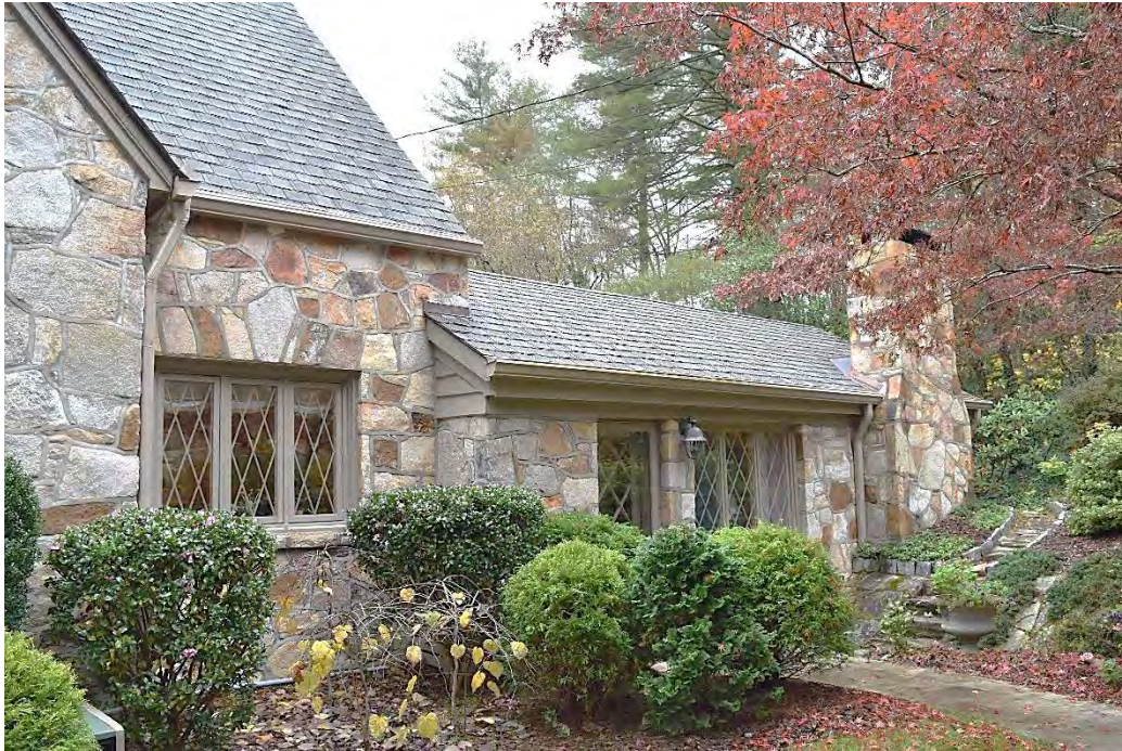
Anders House, North Wing Addition, Façade (East Elevation), Looking Northwest.
