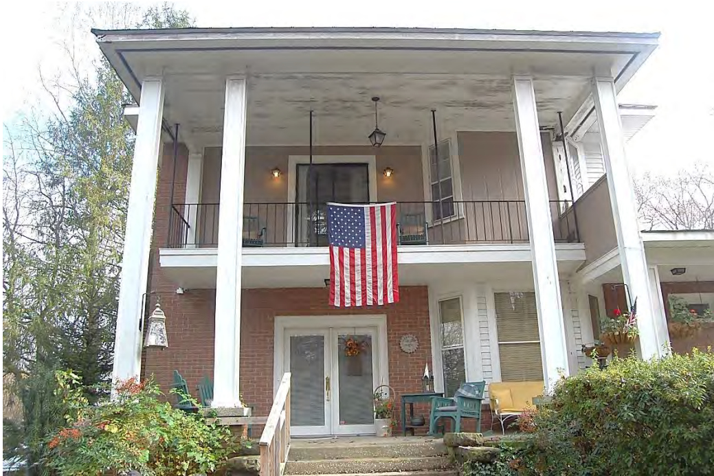
Laughter House, Façade (West Elevation), Looking East.
