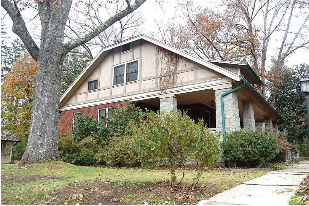
McCall-Malette-Overton House, Side (South) Elevation, Looking North.
