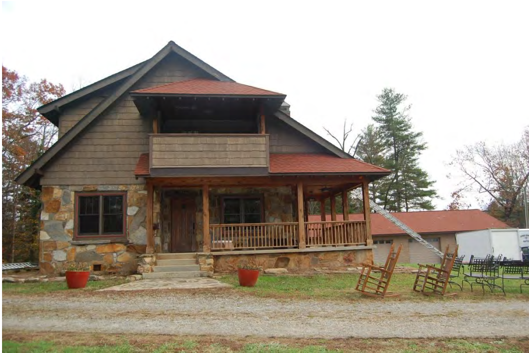
Perry-Harden House, Façade (West Elevation), Looking East. Modern Garage in Background.
