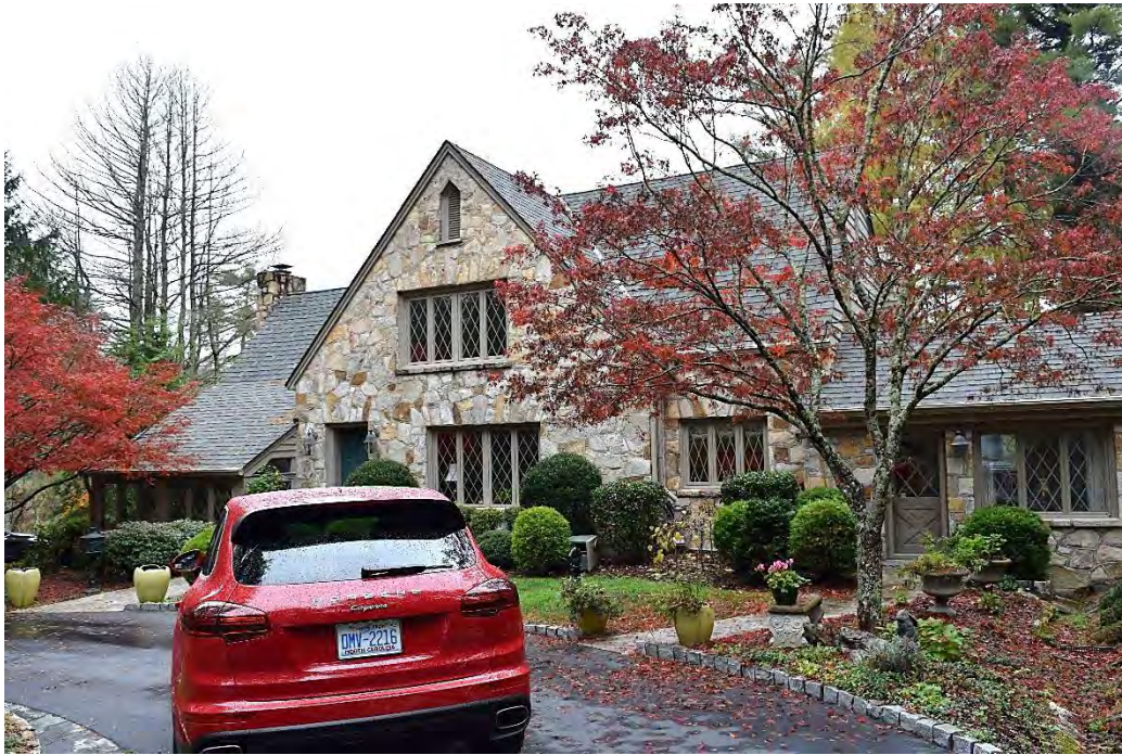
Anders House, Overall View, Looking Southwest.
