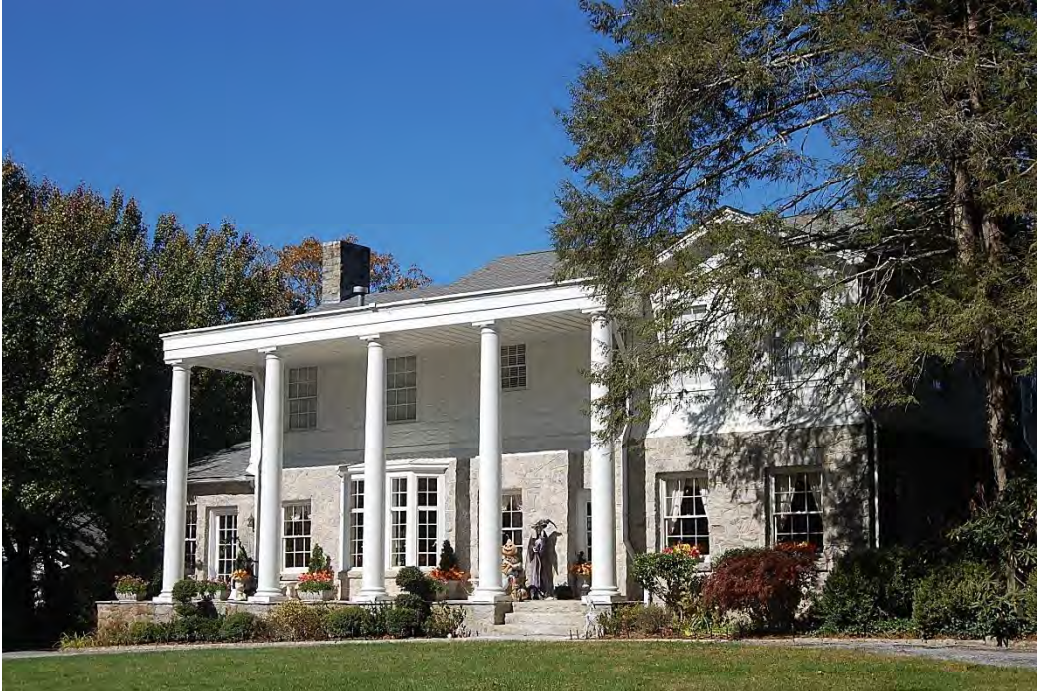
Pinebrook, 2701-03 Kanuga Road, Flat Rock Historic District, Looking West.
