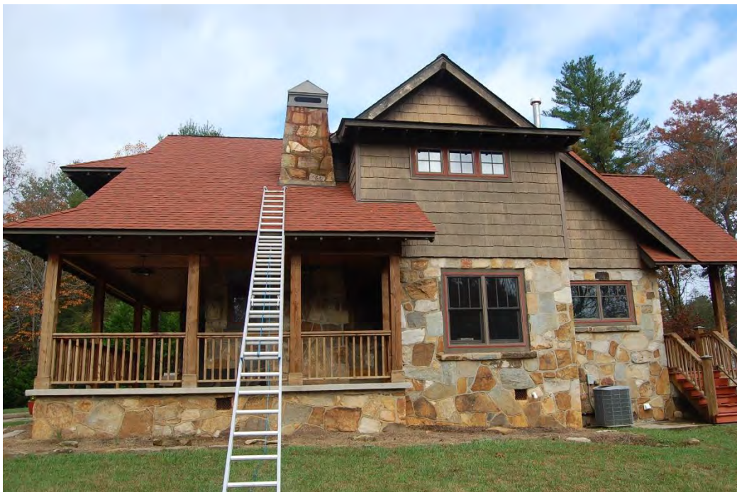
Perry-Harden House, Side (South) Elevation, Looking North.
