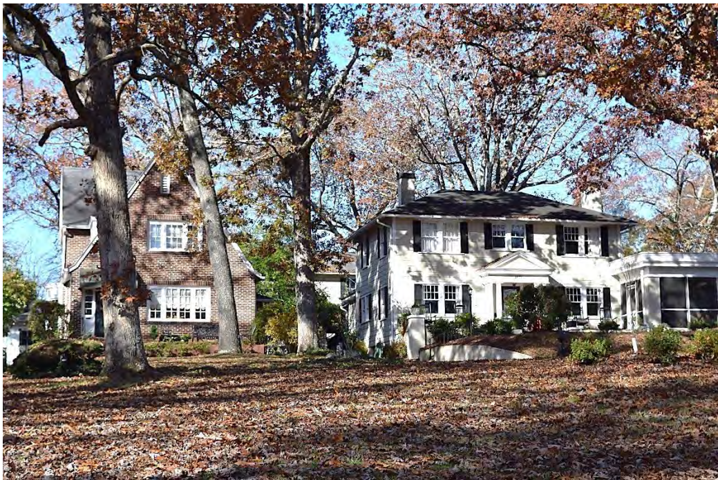
Forest V. Hunter House (ca. 1925), 1615 Druid Hills Avenue (Right) and the Adjacent Colonial Revival Richard Clark House, Hendersonville, Druid Hills Historic District.
