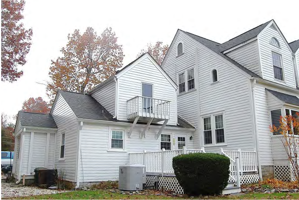
Hayne-Braznell House, Rear (West) and Side (North) Elevations (Right) and Servants' Quarters (Left), Looking East.
