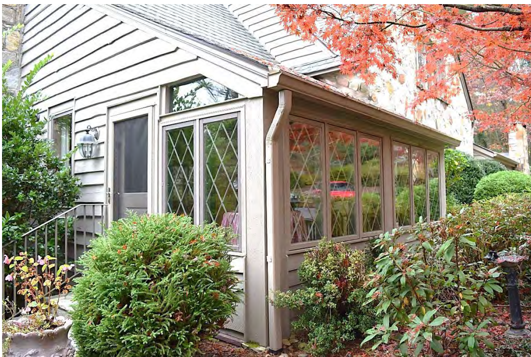
Anders House, South Wing, Front (East) and Side (South) Elevations, Looking Northwest.
