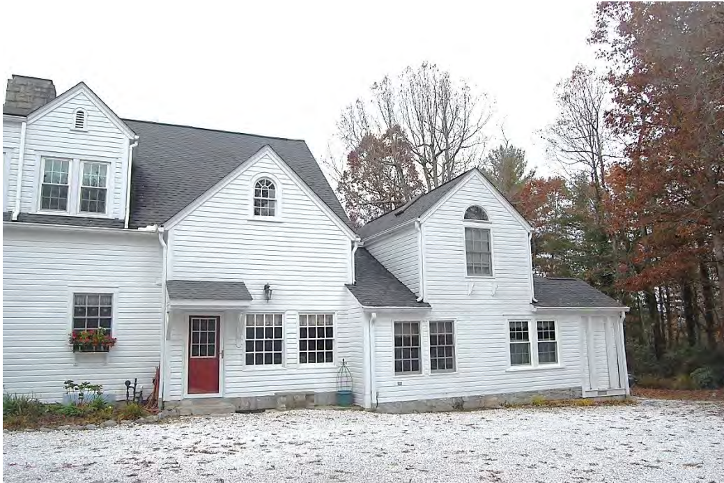
Hayne-Braznell House, Main House, Façade (Left) and Servants' Quarters (Right), Looking Northwest.
