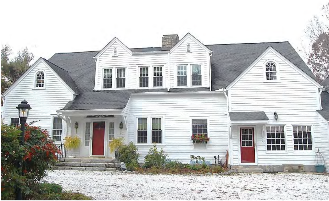
Hayne-Braznell House, Main House, Façade (East Elevation), Looking West.
