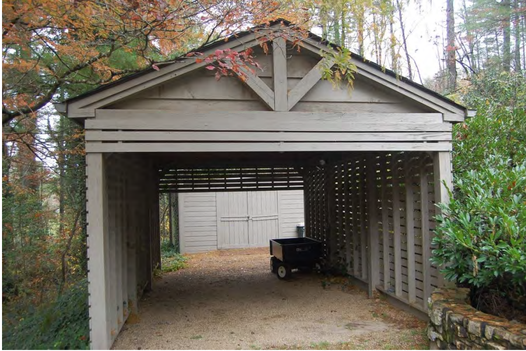
Anders House, Modern Carport and Original Garage (in Rear), Looking Northwest.
