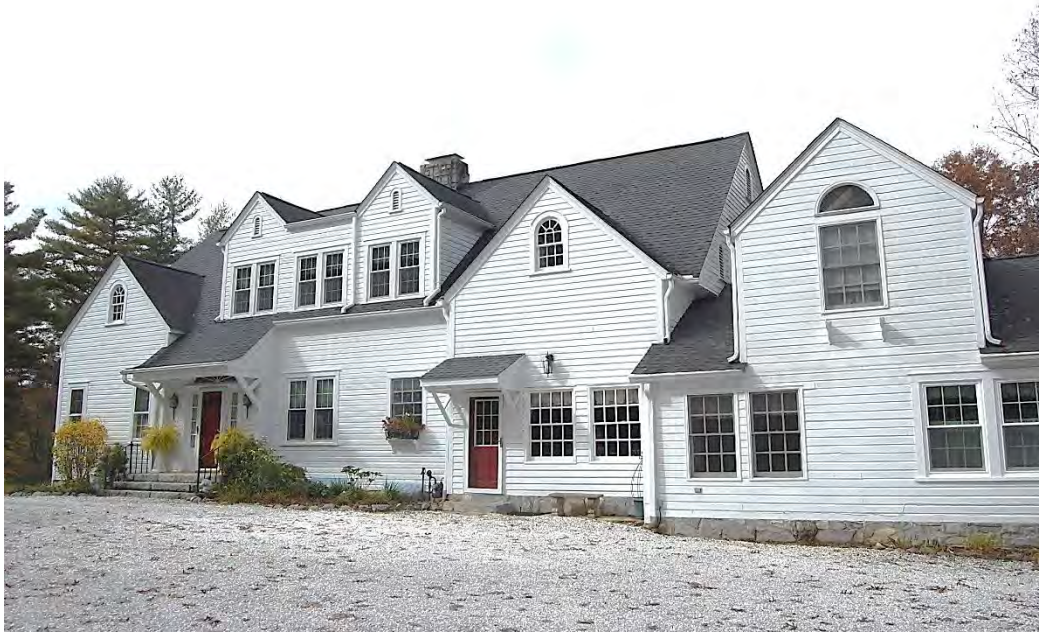
Hayne-Braznell House, Overall View of Façade (East Elevation), Looking West.
