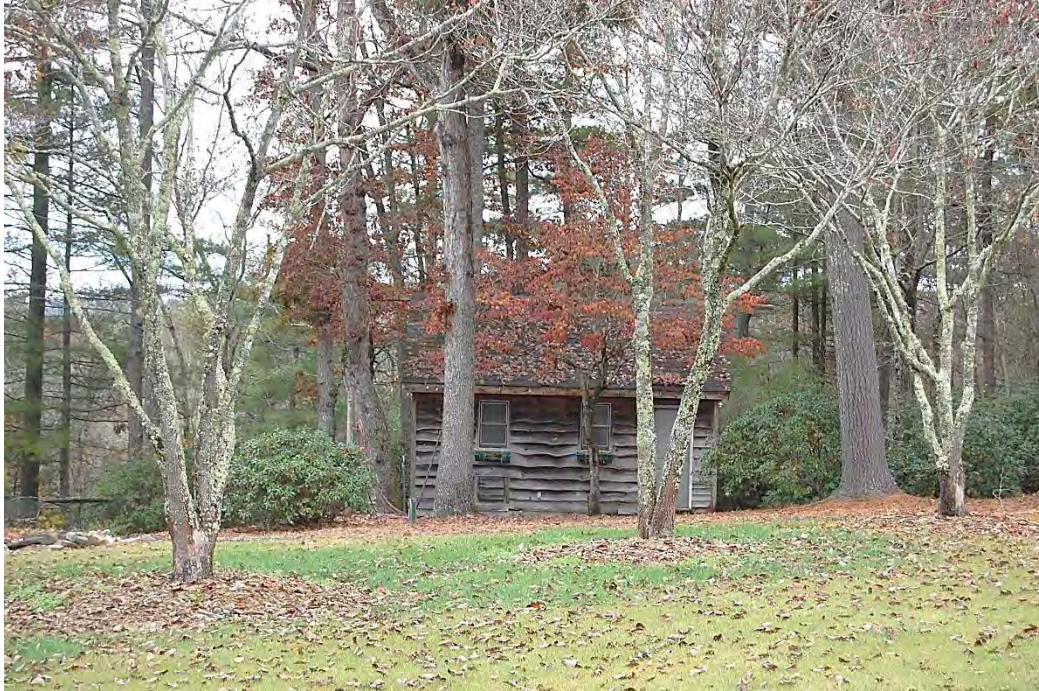
Hayne-Braznell House, Play House/Storage Building, Looking Northwest.
