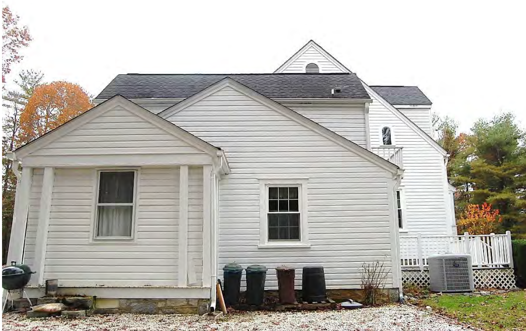
Hayne-Braznell House, Servants' Quarters, North Elevation and Enclosed Porch, Looking South.
