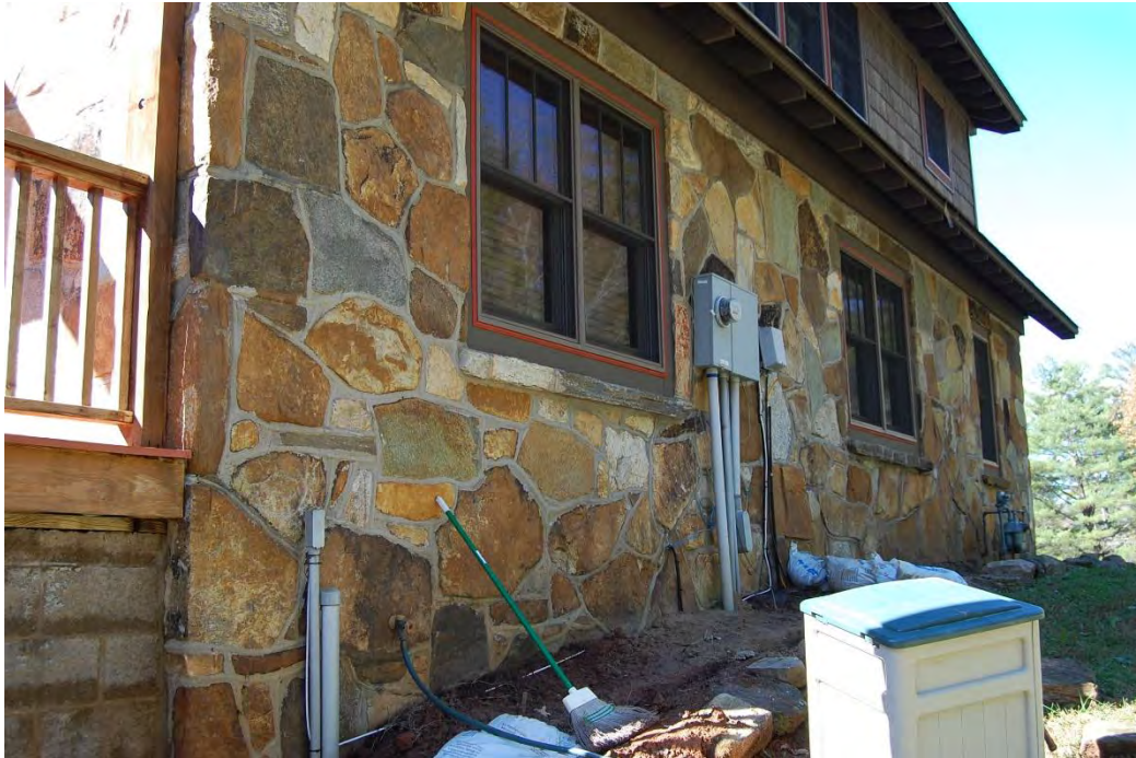
Perry-Harden House, Side (North) Elevation, Looking Southwest.
