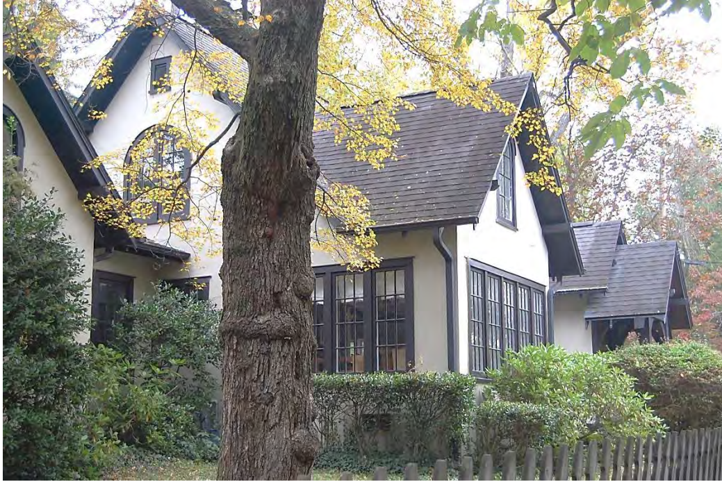
Ray R. Arledge House (ca. 1925), 525 Ehringhaus Street, Hendersonville, West Side Historic District.
