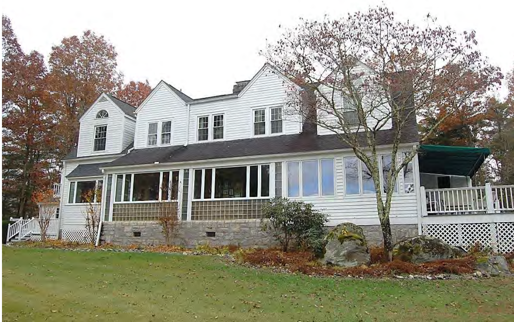
Hayne-Braznell House, Rear (West) Elevation, Looking East.
