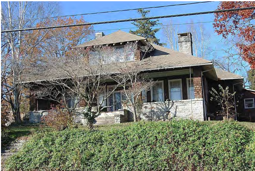
Konsler House (1907), 805 Oakland Street, Hendersonville.
