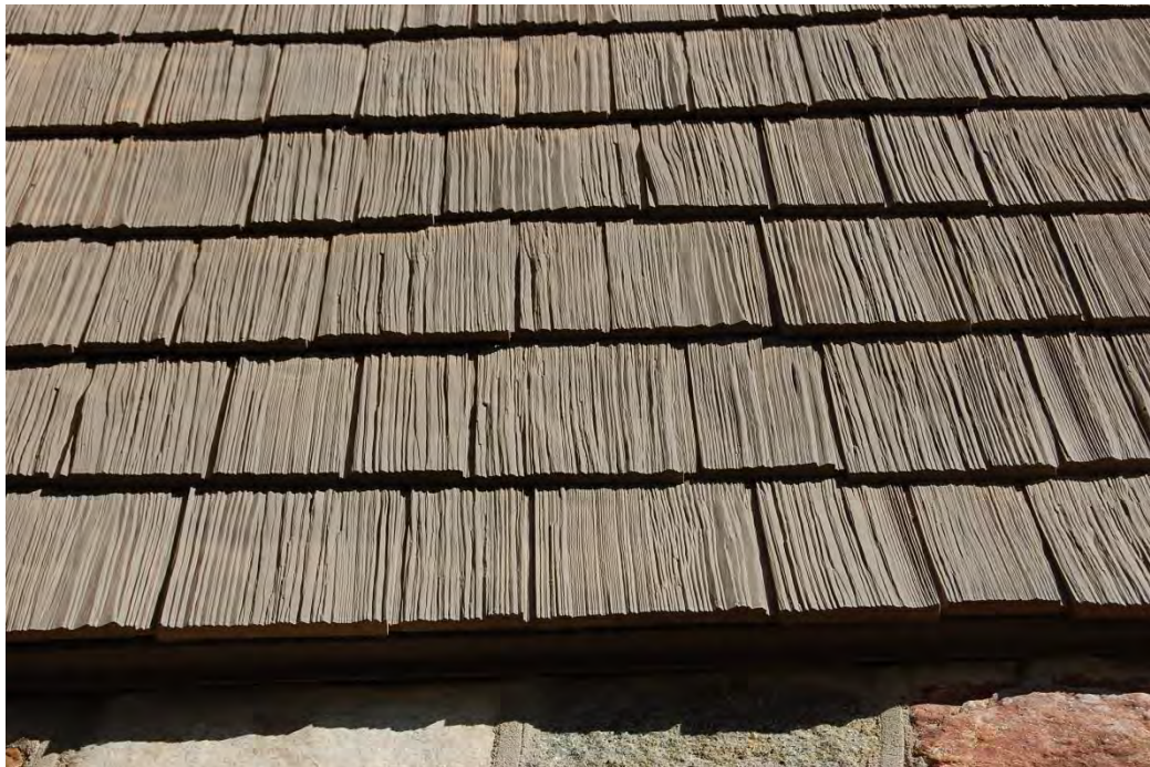
Perry-Harden House, Detail of Modern Shingles, South Elevation.
