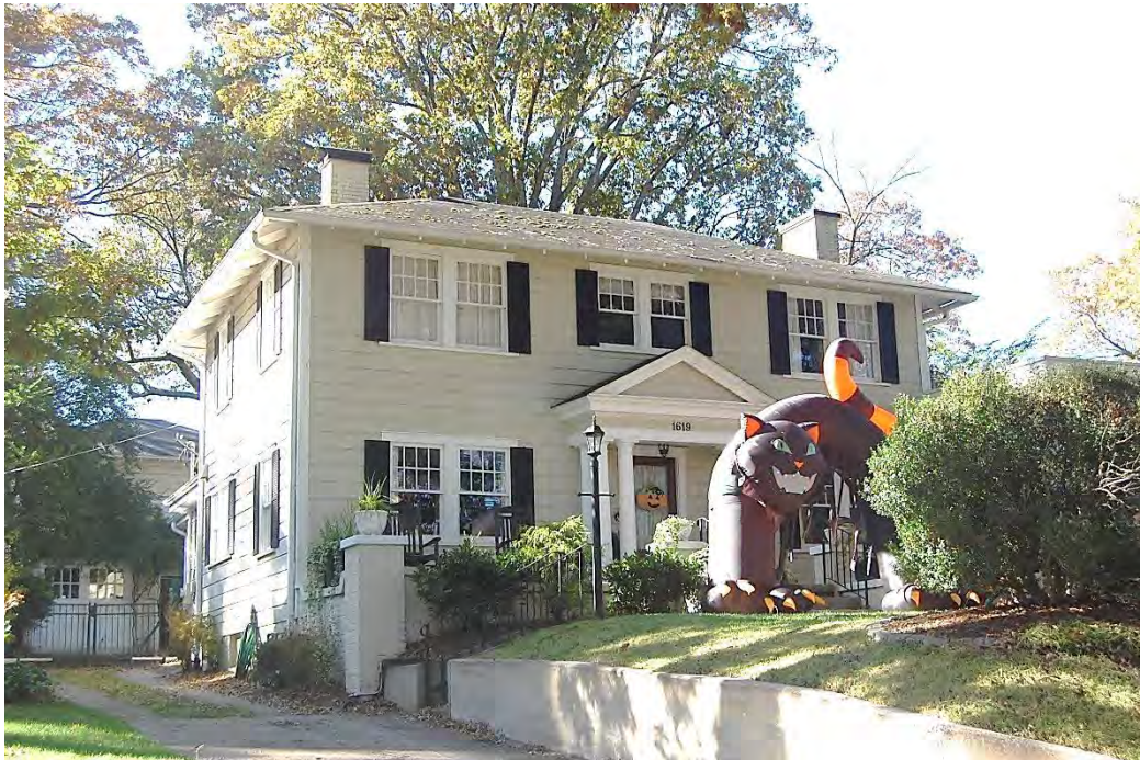
Richard Clark House (ca. 1925), 1619 Druid Hills Avenue, Hendersonville, Druid Hills Historic District.
