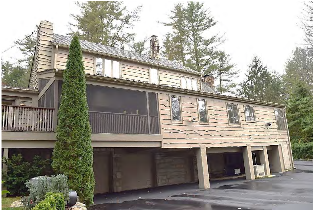
Anders House, Rear (West) Elevation and Modern Rear Addition, Looking Southeast.
