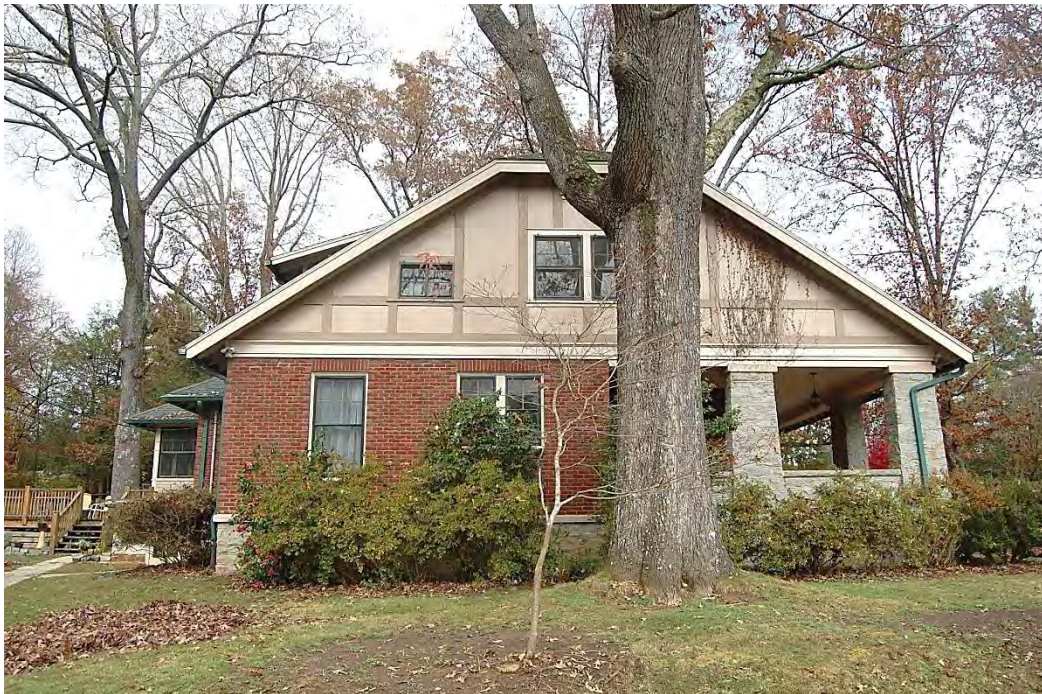
McCall-Malette-Overton House, Side (South) Elevation, Looking North.
