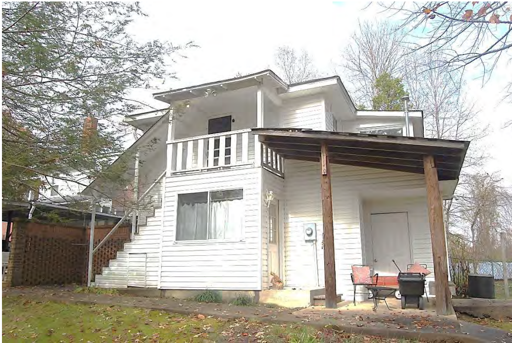
Laughter House, Workshop, South Elevation, and Carport (Left), Looking North.
