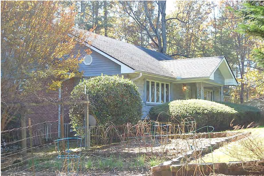
House, 3002 Kanuga Road, Flat Rock Historic District, Looking South.
