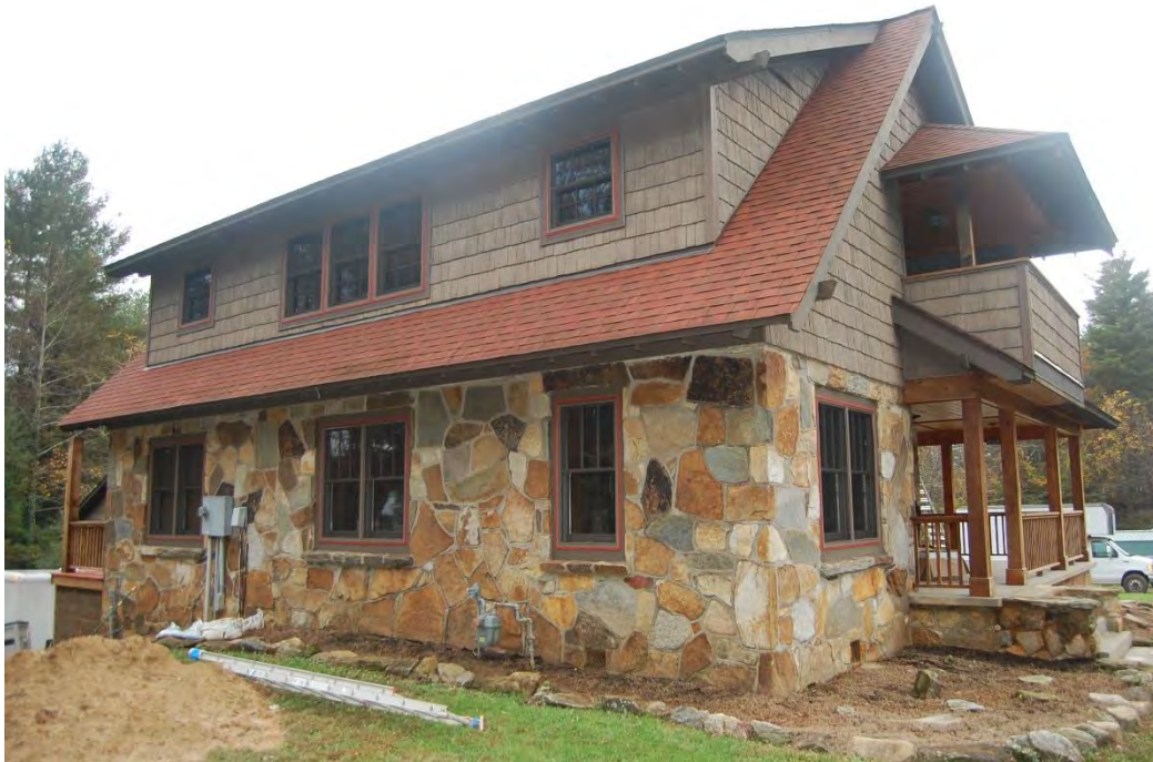
Perry-Harden House, Side (North) Elevation, Looking South.
