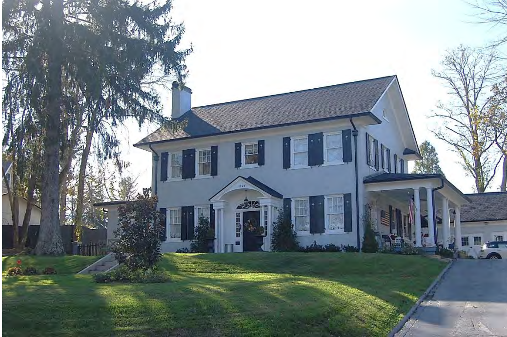
Dr. Robert Sample House (1926), 1125 Highland Avenue, Hendersonville, Hyman Heights Historic District.
