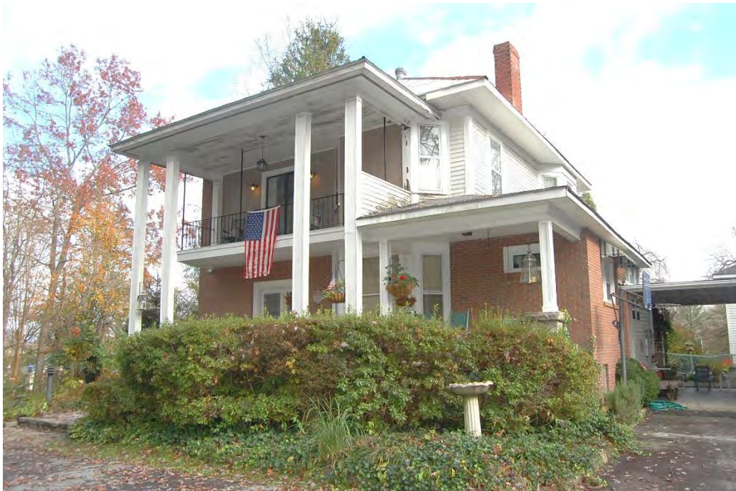
Laughter House, Façade (West Elevation) and Side (South) Elevation, Looking East.
