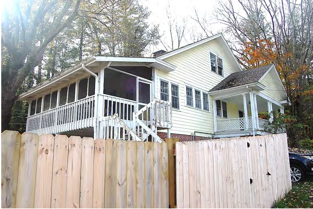
Dominic Podesta House, Rear (West) and Side (North) Elevations, Screened Porch, Looking Southeast.
