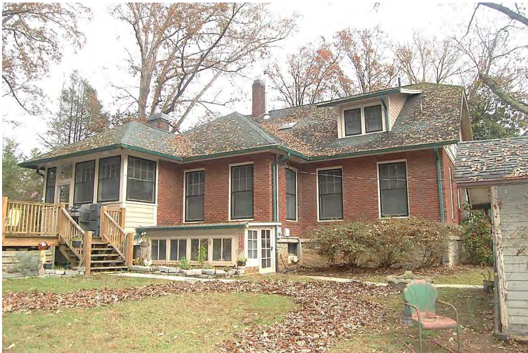
McCall-Malette-Overton House, Rear (West) Elevation, Looking East.
