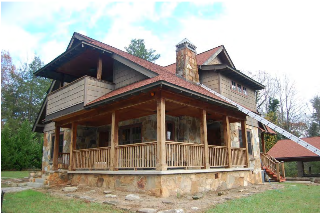
Perry-Harden House, Façade (West Elevation) and Side (South) Elevation, Looking Northeast.
