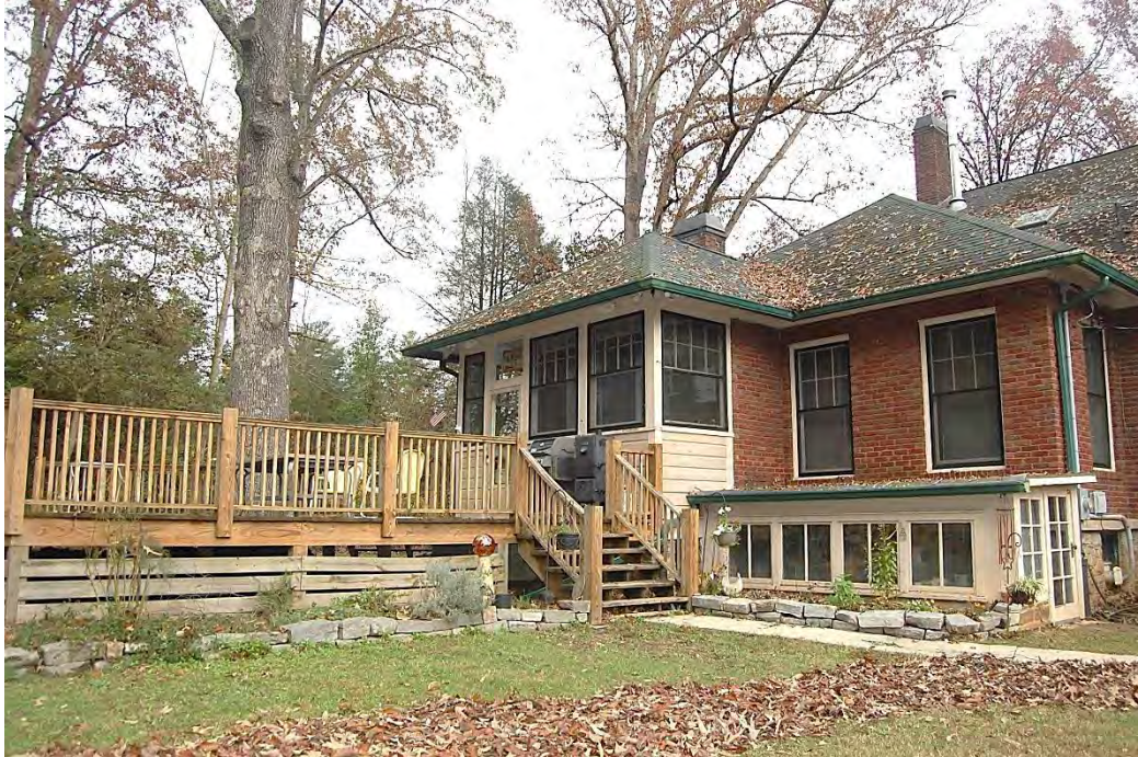
McCall-Malette-Overton House, Rear (West) Elevation, Looking Northeast.
