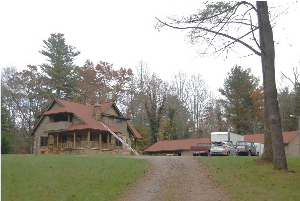
Perry-Harden House, Overall View of House and Setting, Looking Northeast From Kanuga Road. Modern Equipment Storage Building in Background.
