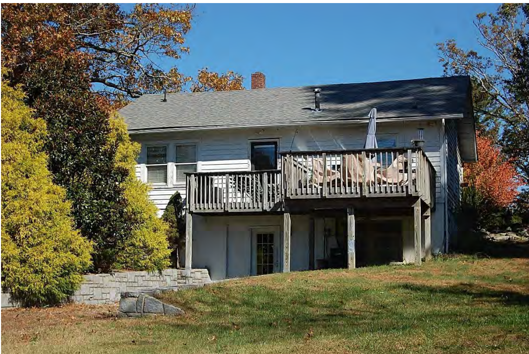
Caretaker's House, Pinebrook, Flat Rock Historic District, Looking North.
