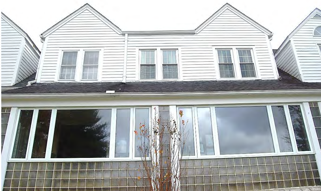
Hayne-Braznell House, Rear (West) Elevation, Porch and Dormer, Looking East.
