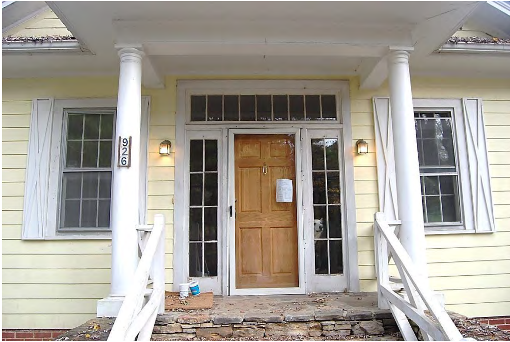
Dominic Podesta House, Façade (West Elevation), Main Entrance, Looking East.
