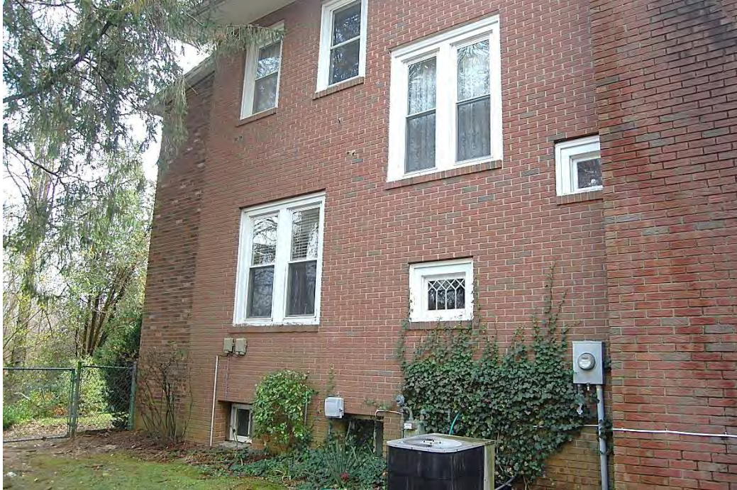
Laughter House, Side (North) Elevation, Looking Southeast.
