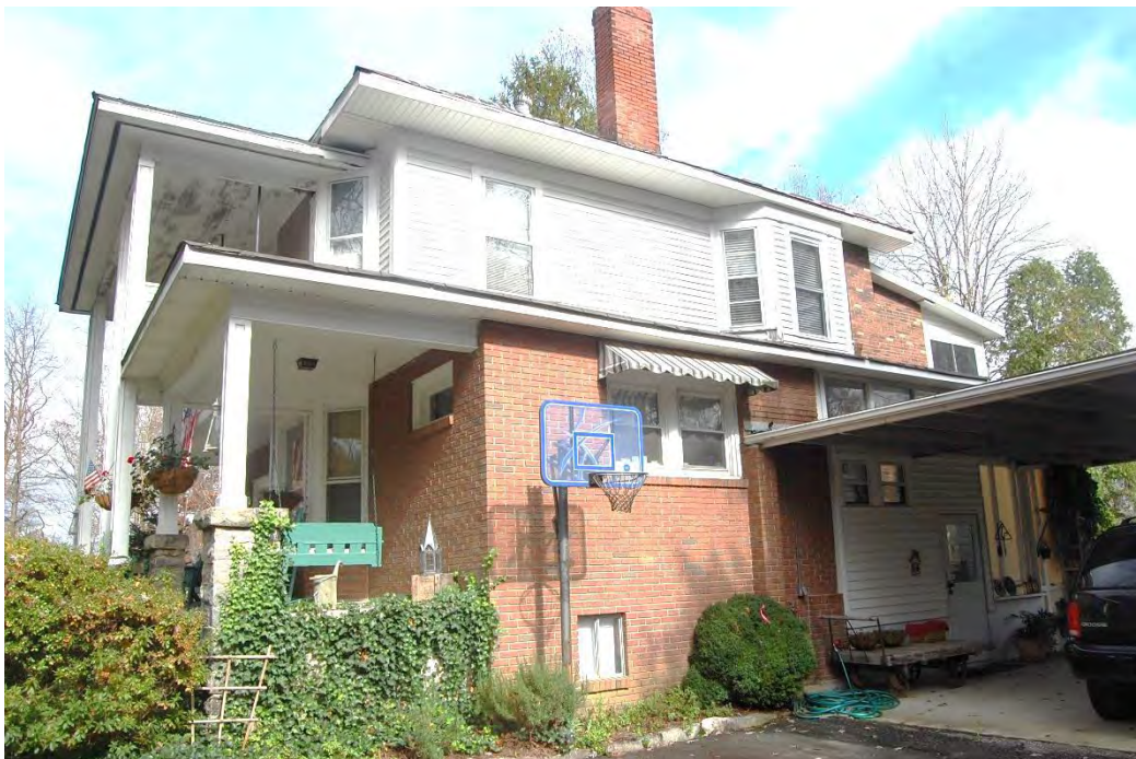
Laughter House, Side (South) Elevation, Looking North.
