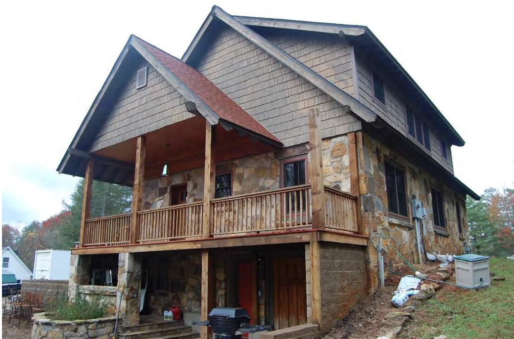
Perry-Harden House, Rear (East) Elevation, Looking West.
